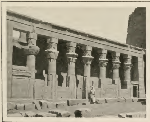
FIG. 432.—EAST FAÇADE OF THE MAMMISI AT PHILÆ. (Phot. Fiorelli.)
